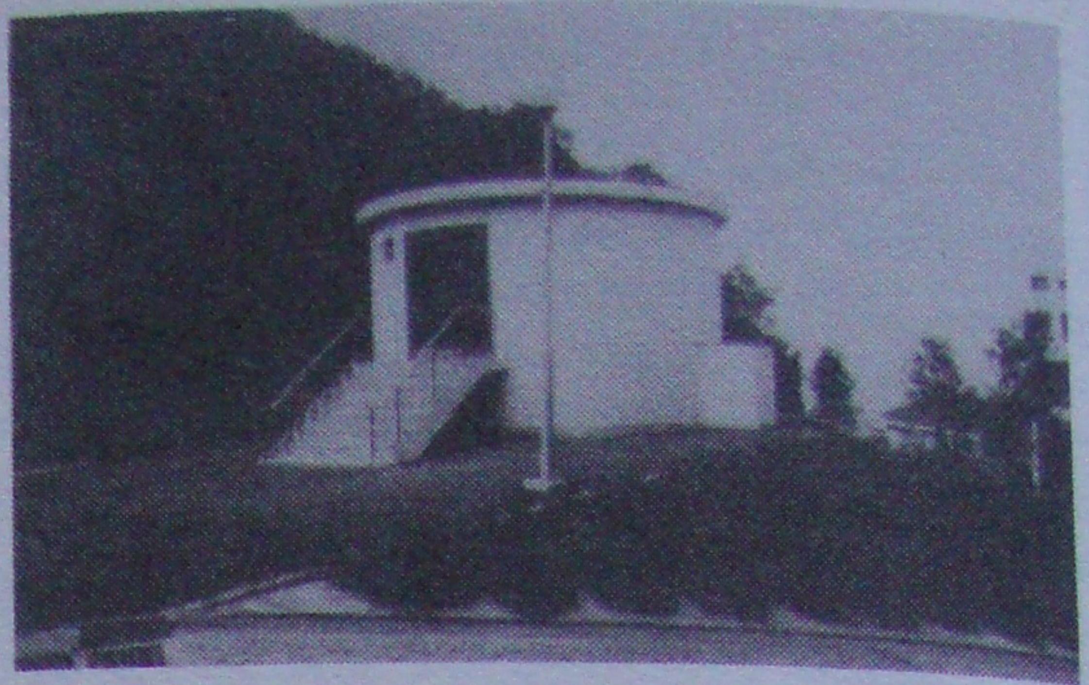
Photo 2 Well for emergency use
