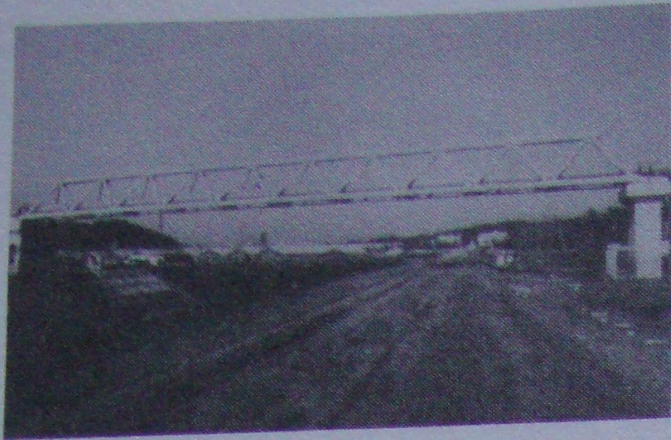
Photo 1 Renewed water piping bridge
